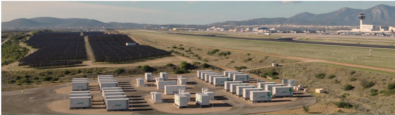
Athens International Airport—The World’s Largest Airport with Integrated Photovoltaic and Energy Storage Location: Athens, Greece Configuration: 123.8 MWh Jinko SunTera liquid-cooled energy storage system, comprising 36 containerized energy storage units Model: Self-generation and self-consumption, with year-round on-site storage and utilization of clean energy
