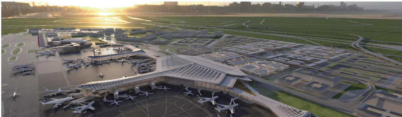
Taiyuan Wuxu Zero-Carbon Airport—China’s First Zero-Carbon Aviation Hub Location: Taiyuan, Shanxi Province, China Configuration: Total installed capacity of 108.5 MW, of which approximately 40 MW consists of Feihu anti-glare modules installed in the light-sensitive areas on either side of the runway Operating model: Self-generation for self-consumption; photovoltaic + medium-to-deep geothermal energy + cross-seasonal heating and cooling storage + multi-form energy storage
