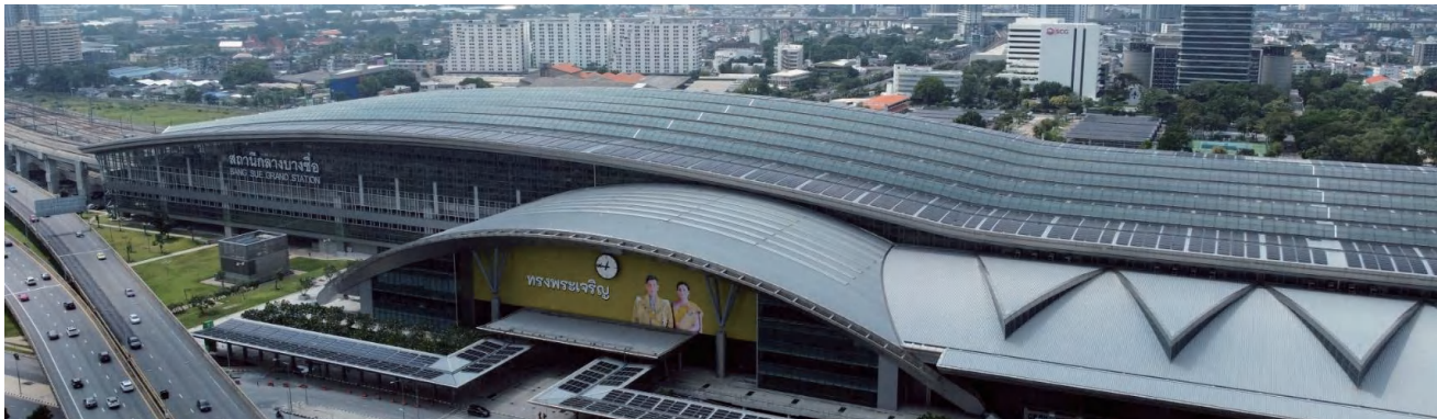
Lumpini Apiva Central Station in Thailand—Thailand’s Largest Rail Hub Location: Bangkok, Thailand Configuration: 9.728 MWp rooftop PV system, featuring over 15,000 Tiger Neo series modules Model: Self-generation for self-consumption
